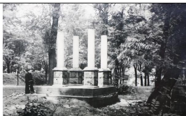
5. The first, demolished in 1955, rosary station in the Katowice-Panewniki Calvary. The Archives of the Franciscan Friars of the Assumption of the Blessed Virgin Mary Province.
