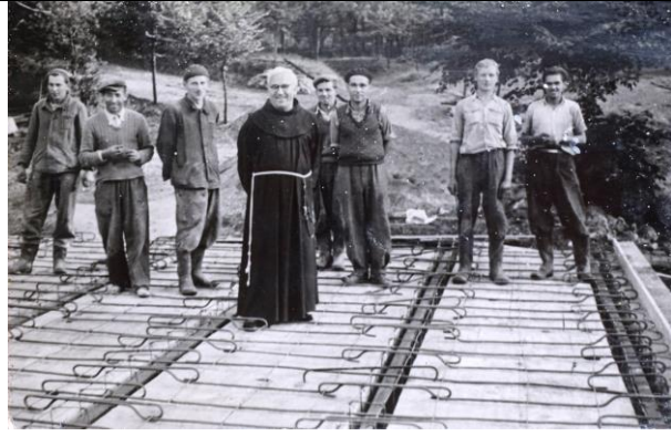
44. Father Norbert Chudoba with workers, on the construction site of the St. Joseph's Bridge on the Calvary in Katowice-Panewniki, 1960. The Archives of the Franciscan Friars of the Assumption of the Blessed Virgin Mary Province.
