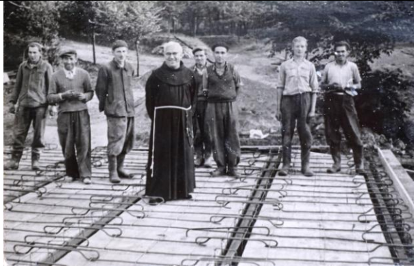
44. Father Norbert Chudoba with workers, on the construction site of the St. Joseph's Bridge on the Calvary in Katowice-Panewniki, 1960. The Archives of the Franciscan Friars of the Assumption of the Blessed Virgin Mary Province.
