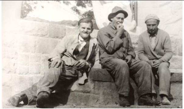
45. Workers on the construction of chapels, 1959. The Archives of the Franciscan Friars of the Assumption of the Blessed Virgin Mary Province.
